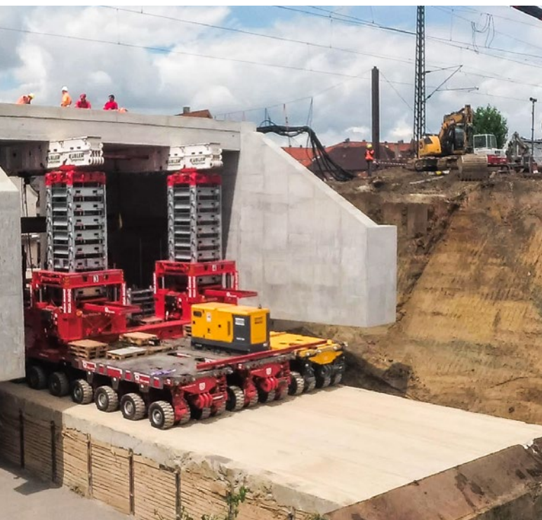
In the dynamic load test, the PLTs had to raise the 1250 tonnes all on their own.
