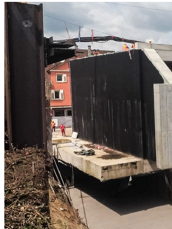
PLTs on SPMTs move prefabricated bridge components weighing up to 1850 tonnes to their final position in their first job.
