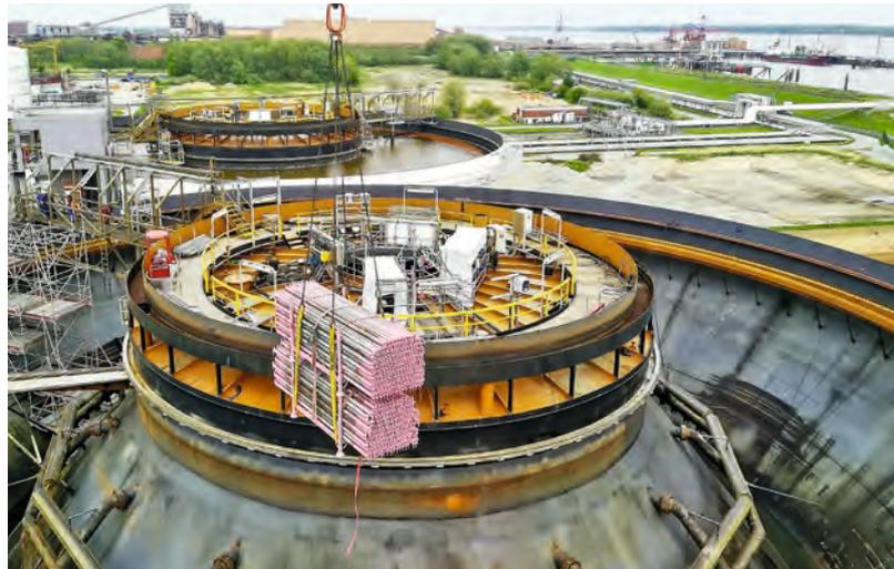
Within four days and three night shifts, the MK 140 lifted a total of 125 tonnes of scaffolding material.
