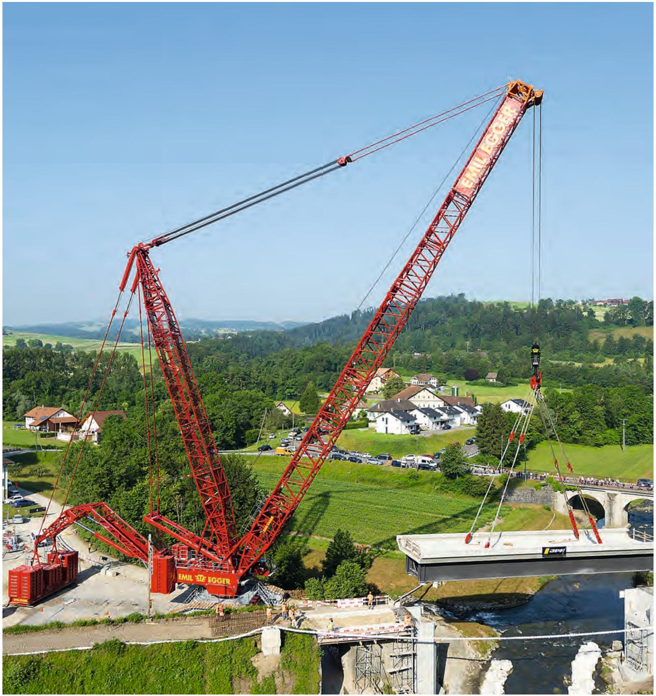
Almost there – the two large hydraulic cylinders extended the derrick ballast to a radius of 28.5 metres for positioning the railway bridge. The maximum possible radius is 30 metres.
