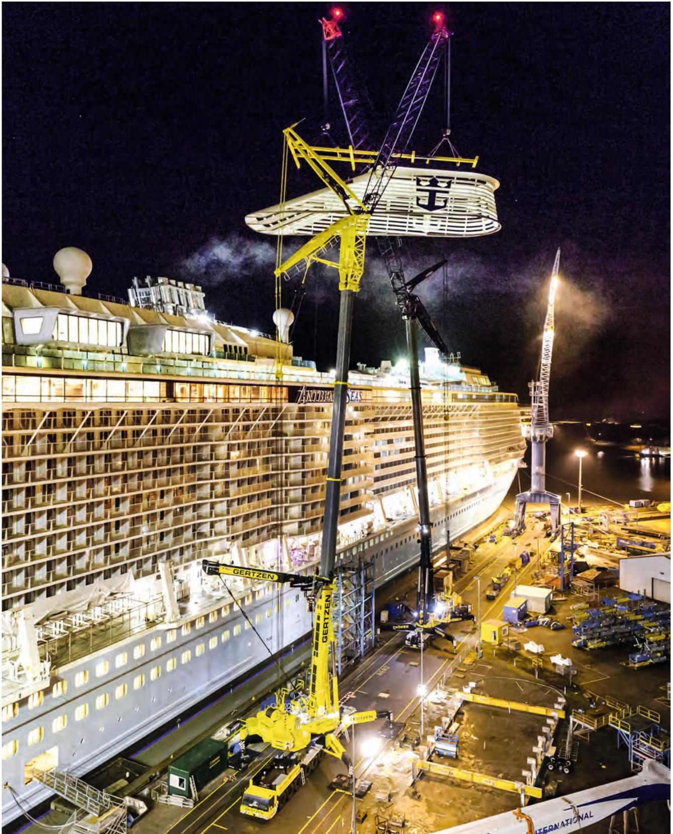
Total precision at night – the two cranes (Thömen and Gertzen) carefully guide the funnel casing between their two luffing jibs.
