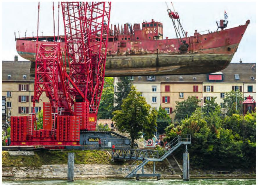
The adjustable ballast allowed the load to be slewed past buildings and obstacles.
