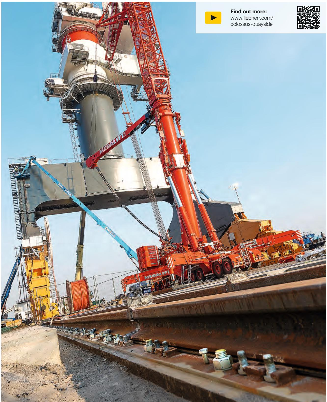
In the future the gantry crane will move on two pairs of the largest available standard rails on a curved section between the northern factory site and the neighbouring quayside – even with loads on the hook. The entire quay had to be rebuilt, including inserting over 600 piles to transfer the immense forces into the foundations.
