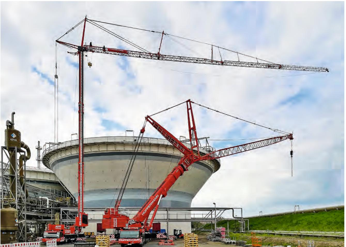
For especially heavy loads, such as the scraper bridges, the mobile construction crane MK 140 was temporarily supported by a Liebherr LTM 1500-8.1 mobile crane.
