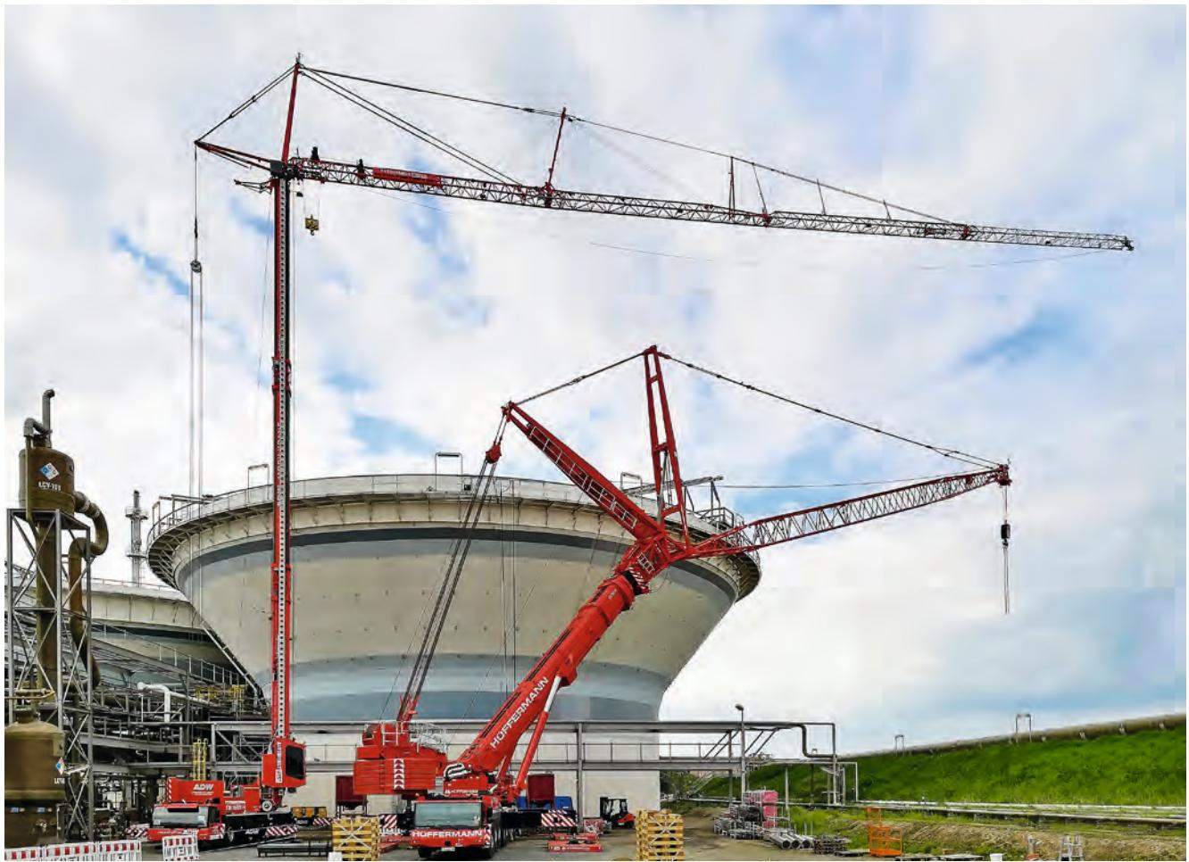
For especially heavy loads, such as the scraper bridges, the mobile construction crane MK 140 was temporarily supported by a Liebherr LTM 1500-8.1 mobile crane.
