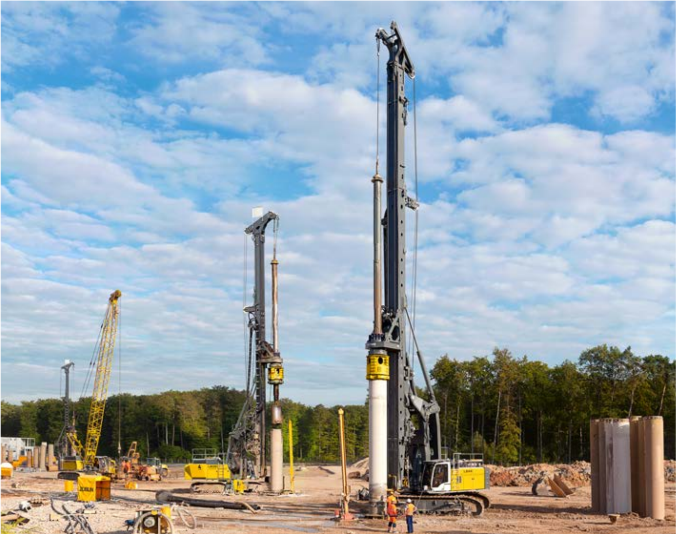
The LB 44 is the largest rotary drilling rig from Liebherr
