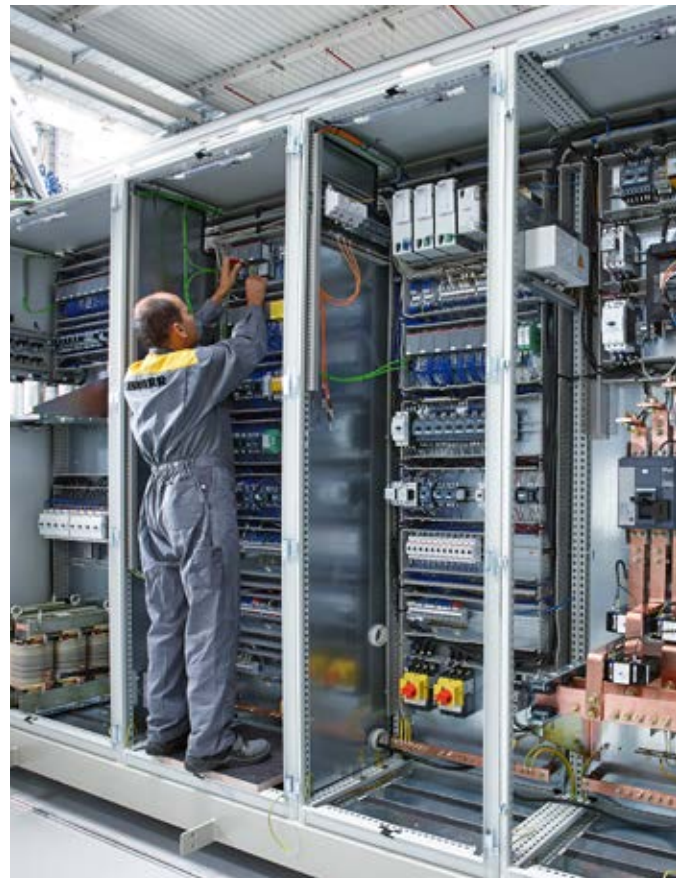
Installation of switchgear for container cranes
