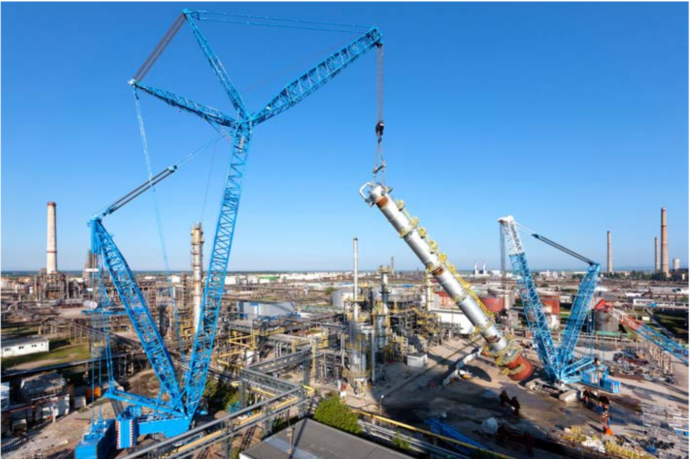
The Liebherr crawler cranes LR 11000 and LR 1750 for tandem lift in Romania
