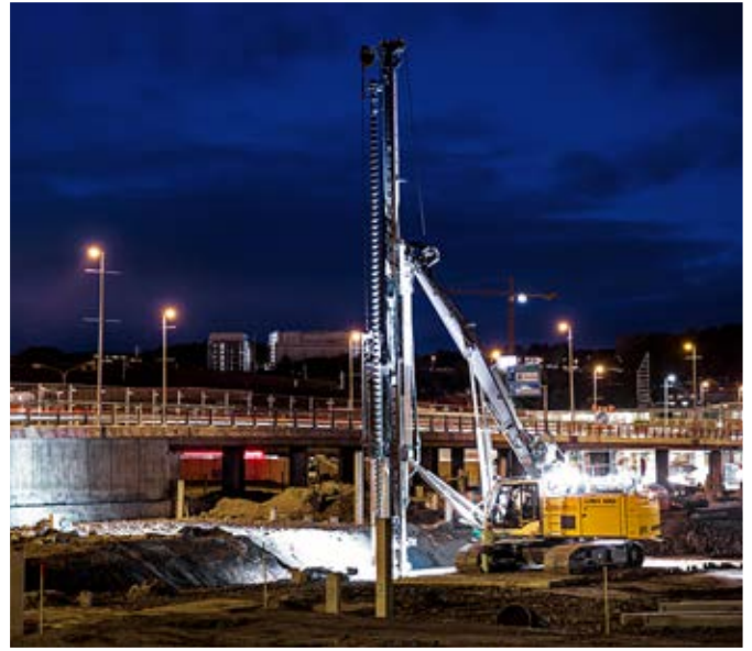
The LRH 100 carrying out piling work in Gothenberg, Sweden
