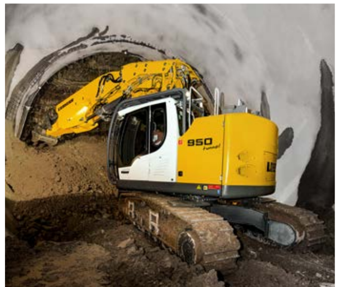
The Liebherr crawler excavator R 950 Tunnel in use in Stuttgart (Germany)
