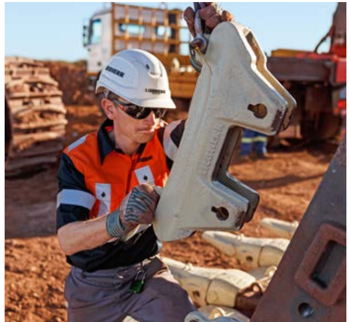
Replacement of Liebherr GET in South Africa
