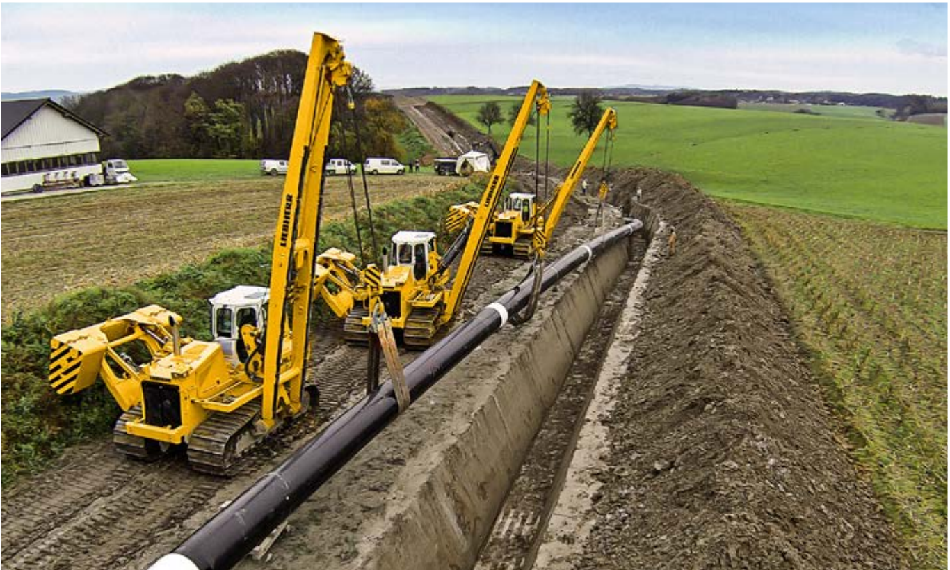
The Liebherr pipe layer in use in Austria
