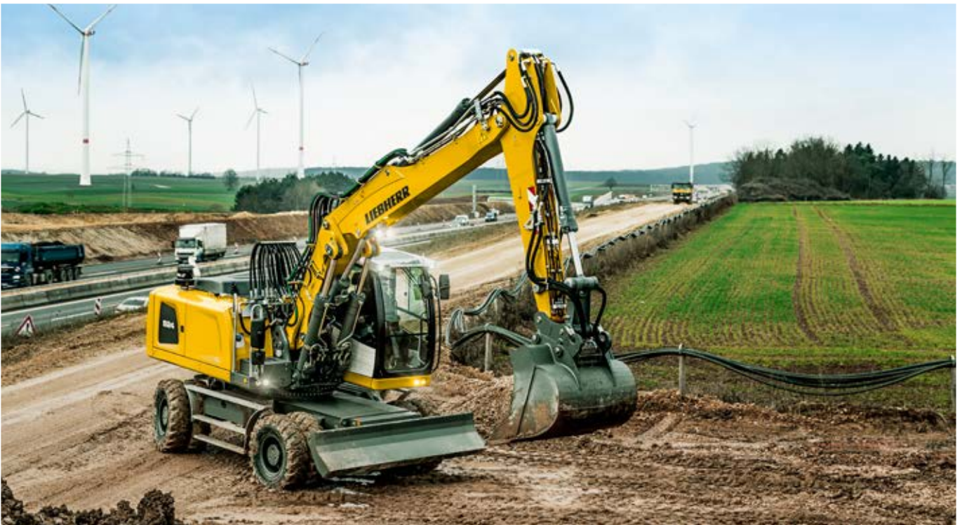
The A 924 Litronic on a motorway construction site in Dornstadt (Germany)
