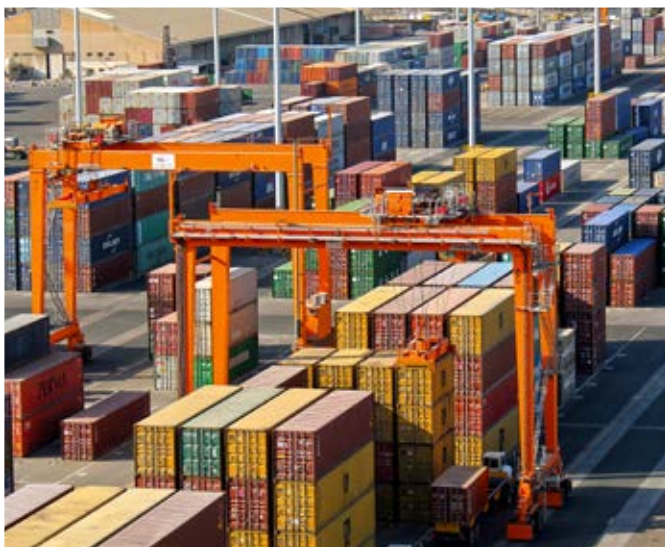
Two Liebherr rubber tyre gantry cranes stack containers in the Port of Shuaiba (Kuwait)
