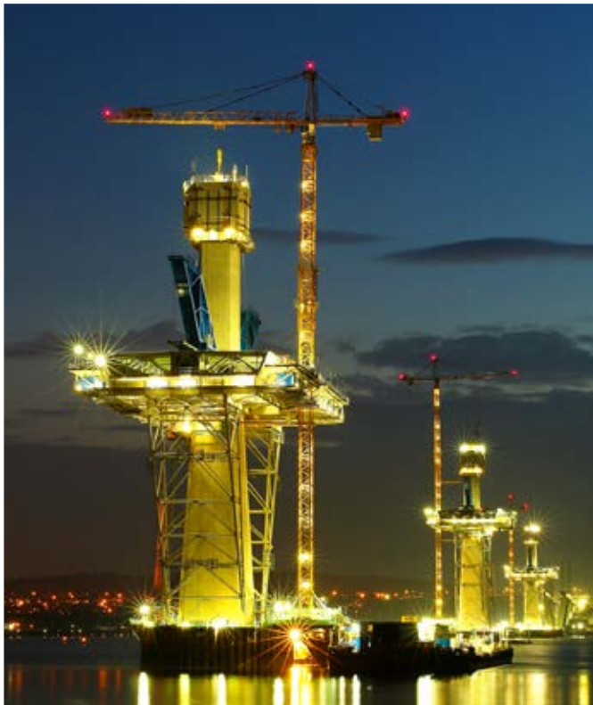
630 EC-H cranes for the construction of Forth Crossing Bridge in Scotland
