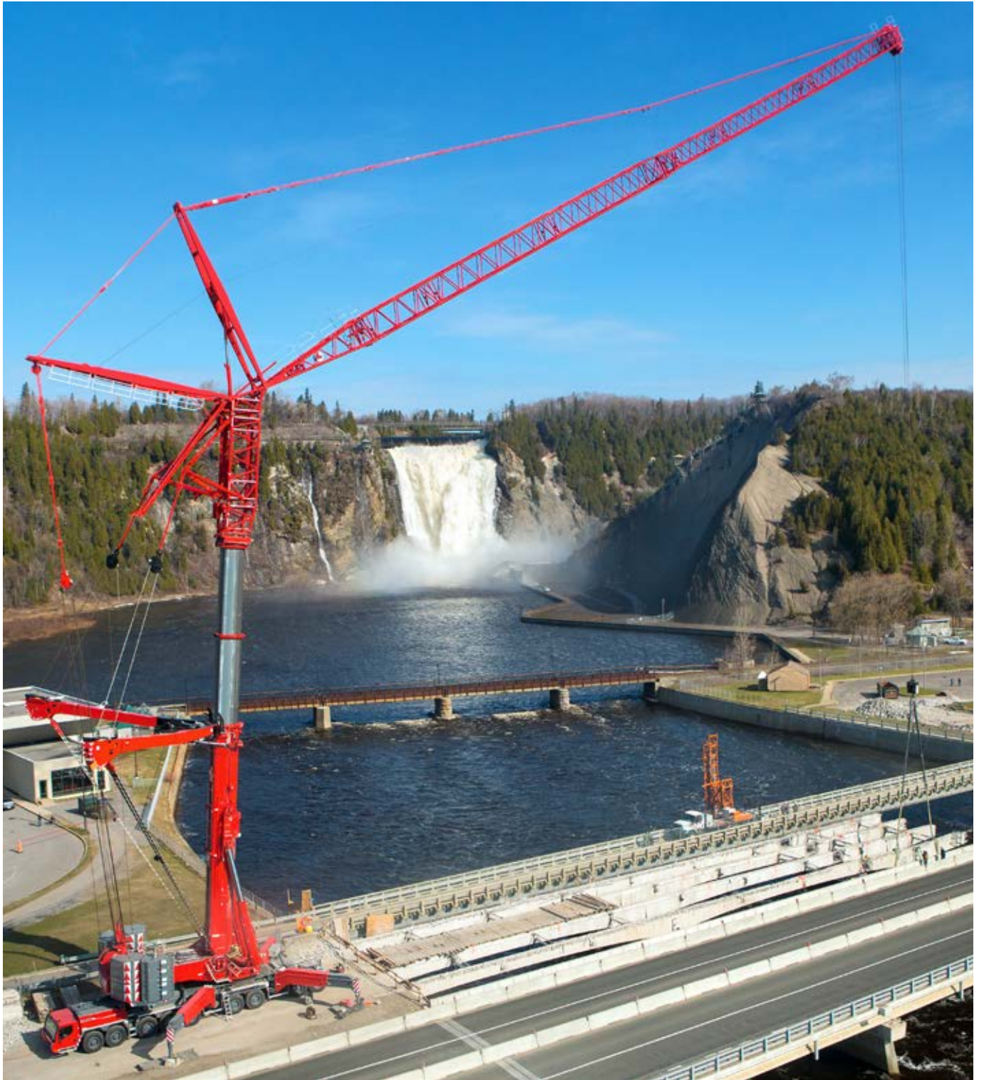
Bridge assembly with a LTM 11200-9.1 in Canada
